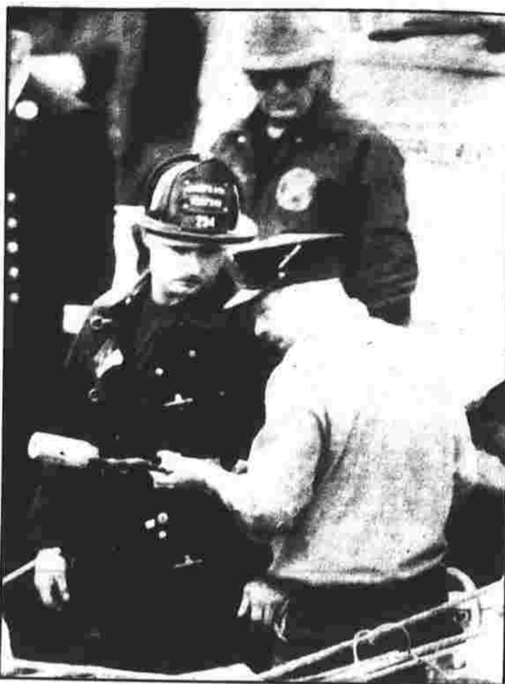
Firefighters prepare to use an electronic device to look for survivors in the rubble of the apartment building under construction in Bridgeport that collapsed Thursday. Another story and picture on page 7.
